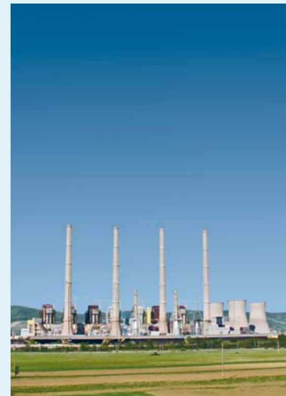
Air Pollution Control technology is an important component to meet strict environmental regulations. This photo shows the turnkey installation of flue gas desulphurization pollution control for a thermal power plant in Romania. ▶
