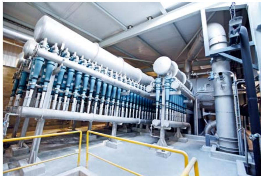
A view of the ANDRITZ FlyingWing Deculator deaeration system with integrated cleaners. ▼
