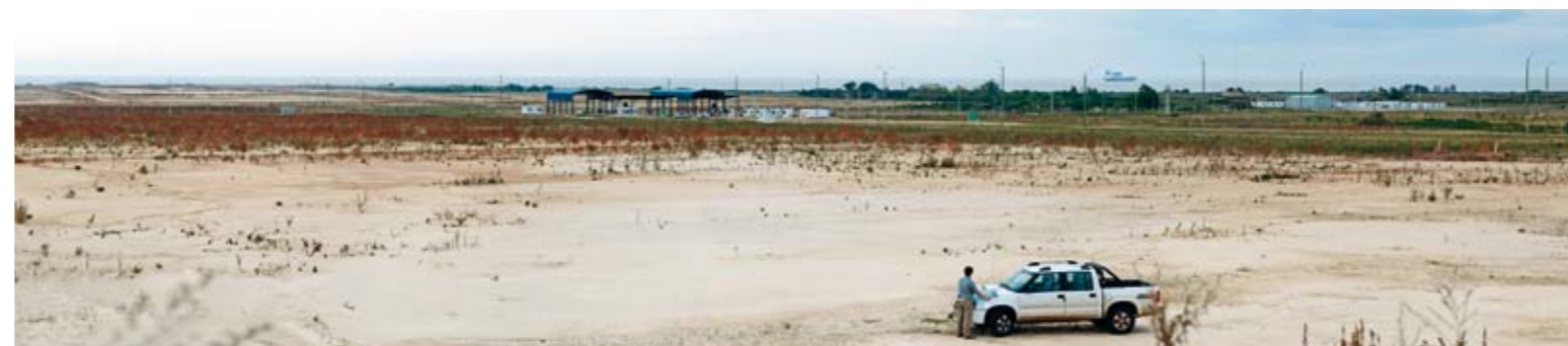
▲ From May 2008 until April 2010, a massive amount of earth was moved, boreholes were drilled for civil works, environmental baselines and approvals were established, even the evaluation and preservation of a wrecked barge in the port area (deemed historically significant) was completed. The site is now ready for ANDRITZ's Uruguayan subcontractors to begin the civil works.
