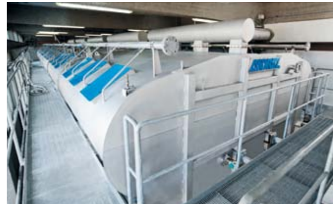
One of the benefits of SelectaFlot is that it is compact, allowing the Lucca mill to save money by lifting the unit into position through second-story openings in an existing building. It was a tight fit. ▶
