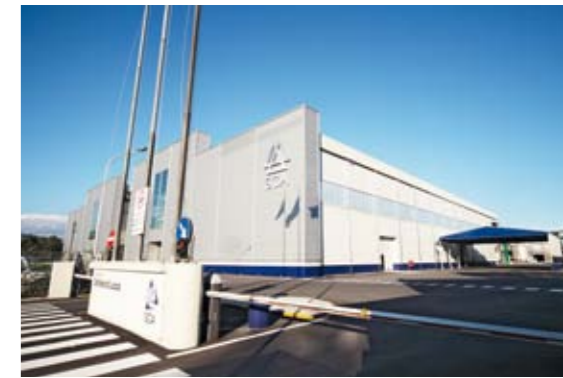
▲ The arrival of the ANDRITZ SelectaFlot unit, a new disc filter, and other stock preparation components marked the decision by SCA Containerboard to improve the quality of the top layer (white top) for PM2 at Lucca.
