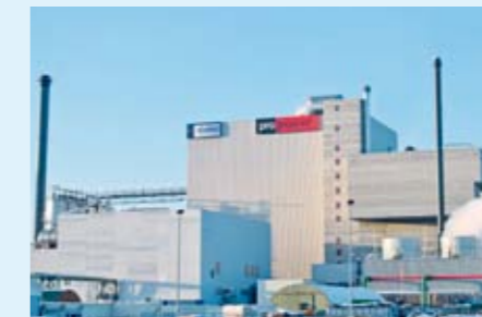
▲ AE&E delivered the world’s largest alternative fuel boiler plant in Eisenhüttenstadt, Germany which provides power and steam for the nearby ProPapier paper mill.
