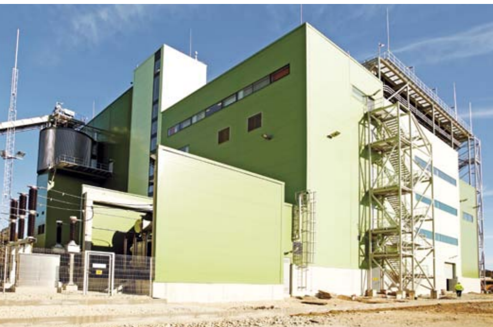
▲ Fortum's CHP plant in Pärnu, Estonia considerably increases energy efficiency and the biomass fuels reduce CO 2 emissions by more than 60%. ▼
