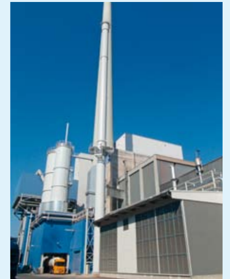
▲ For the growing Waste-to-Power segment, AE&E supplied this fluidized bed boiler firing refuse-derived fuel, with TURBOSORP air pollution control, in Witzhausen, Germany.
